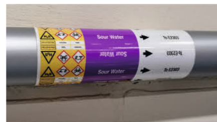
Pipe Marking according ISO 20560-1
